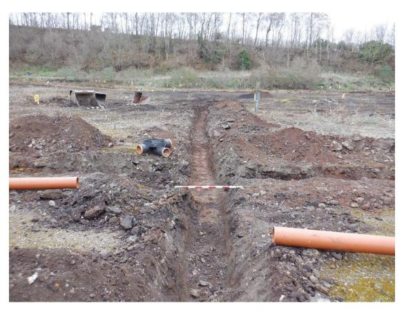
Plate 1. Trenches for pipe runs (looking North)
